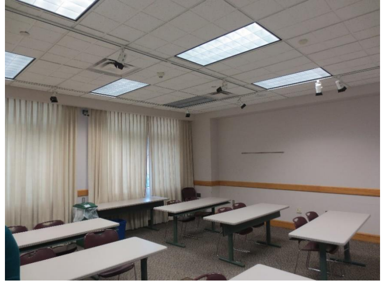
Typical T8 Light Fixtures
